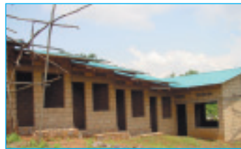
Construction of Kibungo Diocesan Training Centre
